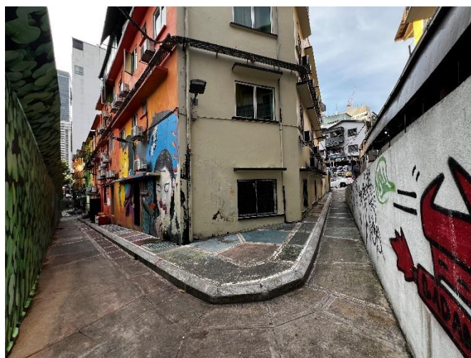
Fig. 7: Kominiti di Alor , lack of maintenance (author,2025)
