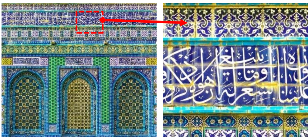
Fig. 5: Faience tilework at the exterior of the dome of the rock in Palestine
