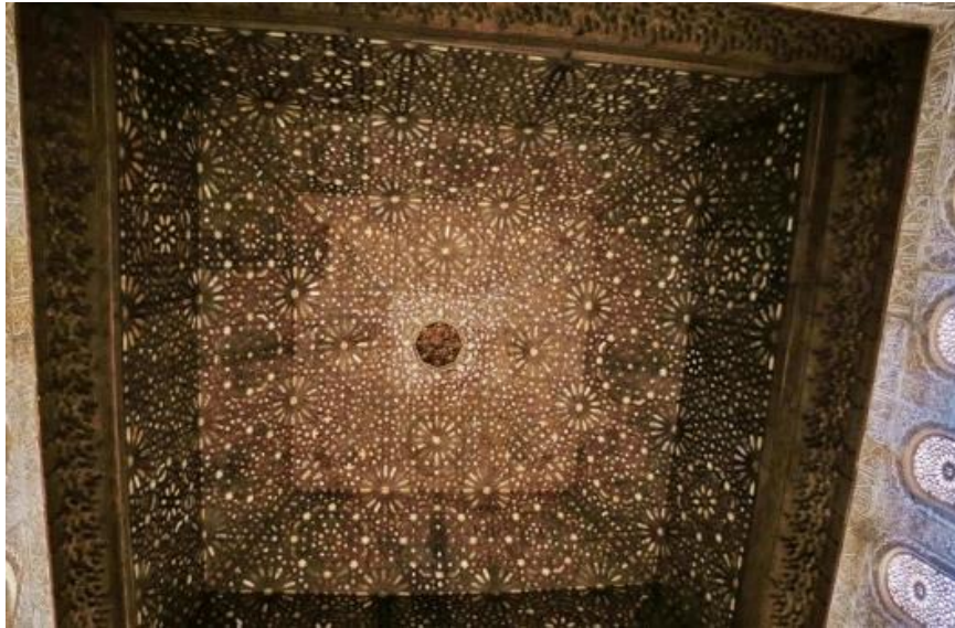
Fig. 17: Intricate wooden ceiling at the hall of the throne in Alhambra palace (Source: lea, 2016)
