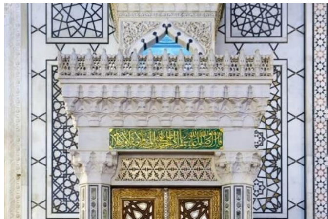
Fig 11: woodwork and decorated Ablaq and marblework (Source: Yagh, 2024)
