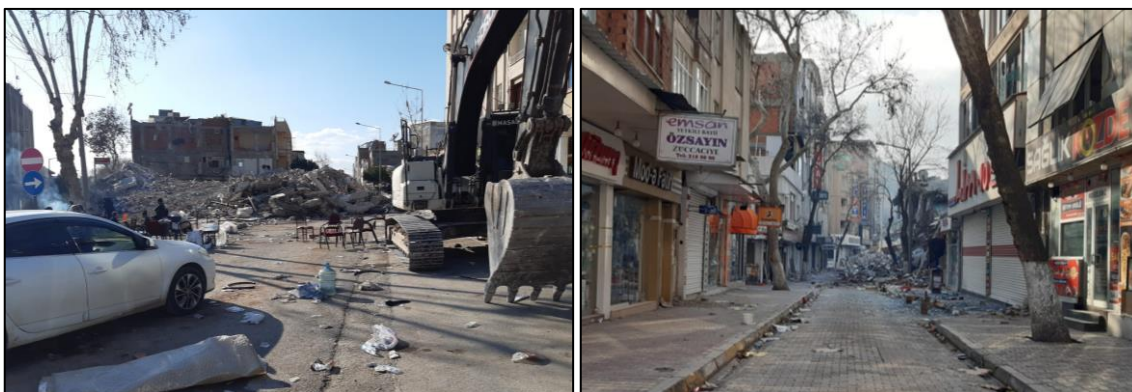
Fig. 2: Blocked roads in Adıyaman after Kahramanmaraş earthquakes in 2023.
