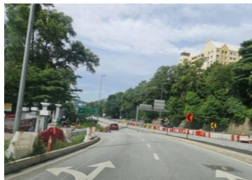
(a) Lack of sidewalk even though the trees and greenery provide enough shade along the street
