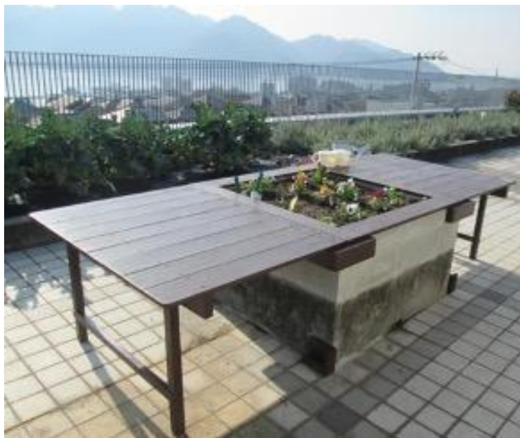
Fig. 5: After implementation, an accessible, structured planter caters to wheelchair users and other disabilities in the TSSG.
