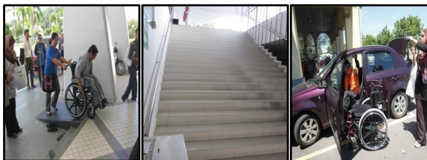
Figure 1, 2 & 3: The entrance of Masjid has many designs and most of the designs are with split level, steps, having series of staircases and some designed with wrong specifications. These are barriers and difficulties faced by the Persons with Disabilities (PwDs) and elderly every single day to go to Masjid and even to perform the obligatory Friday prayer. They usually refuse physical help as they would like to be independent.
