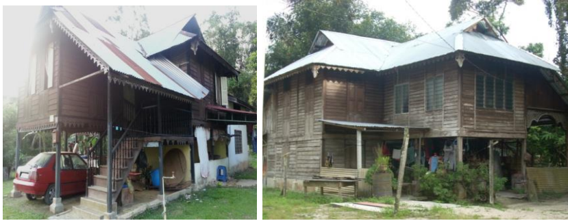
Figure 7: Old traditional Perak houses found in Padang Changkat and Kota Lama Kiri
