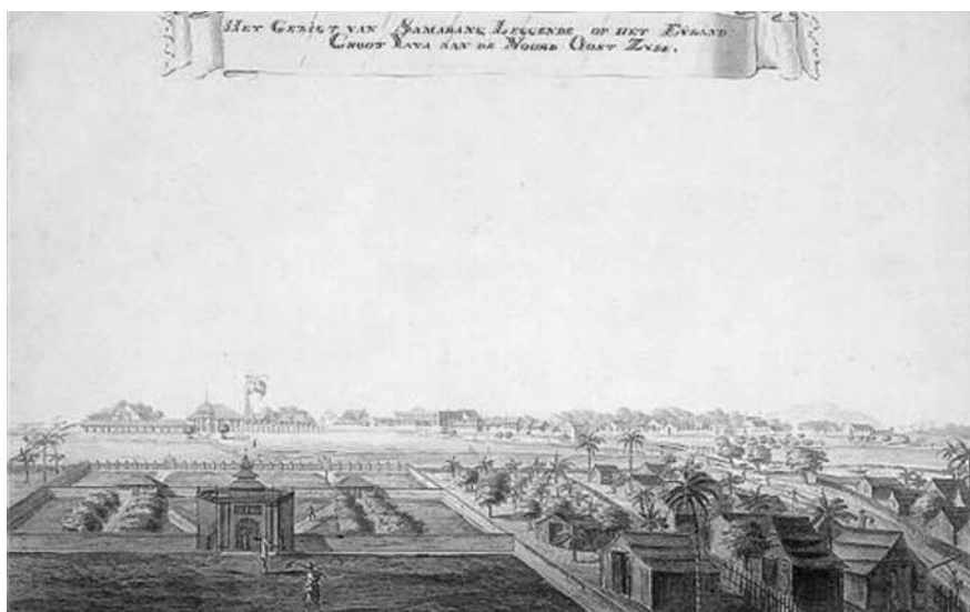
Figure 7 Center of the old city Semarang (Sekayu or Kanjengan ?), the colonial city as the background ( alan Pemuda or Kota Lama?) painted by Johannes Racht (1857). Source: skyscrapercity.com
