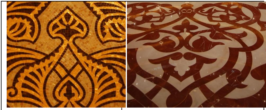
Figure 5. Gold glass mosaic panels and marble inlay flooring—Emirates Palace
