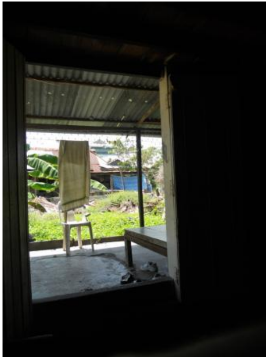
Figure 17: Threshold at front door to prevent water from getting in
