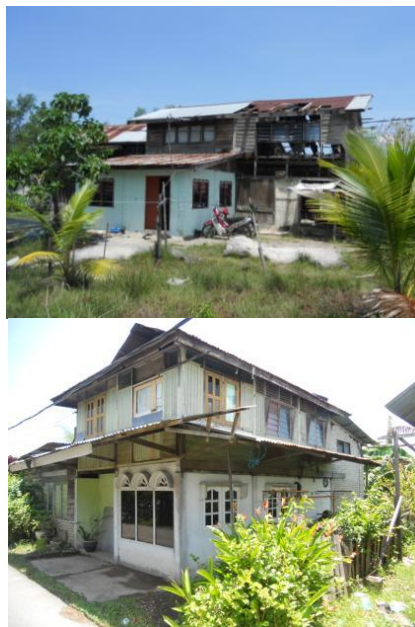
Figure 13: Renovated house that has additional living space on ground floor Source: Author
