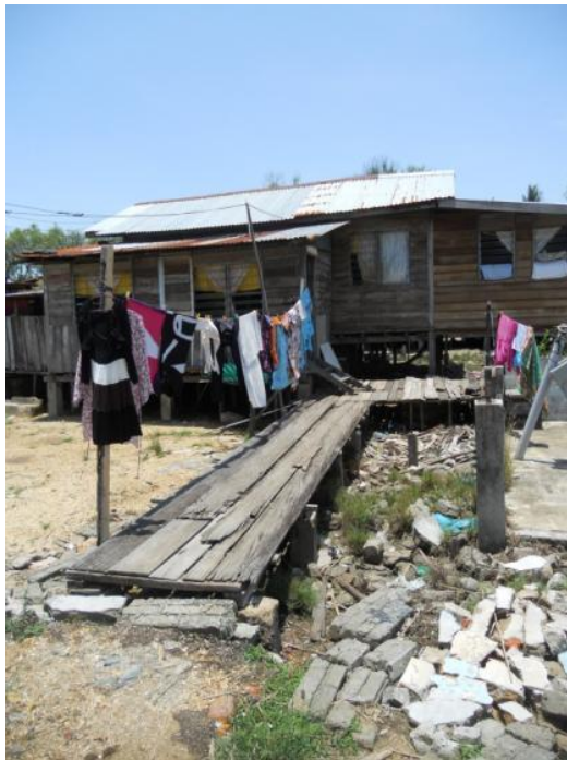
Figure 8: Raised platform as walkway
