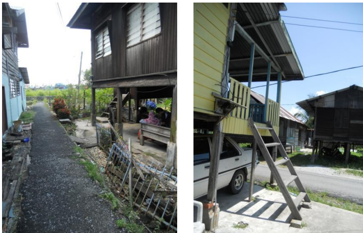
Figure 9: Tar road replaced the use of raised platform Source: Author
