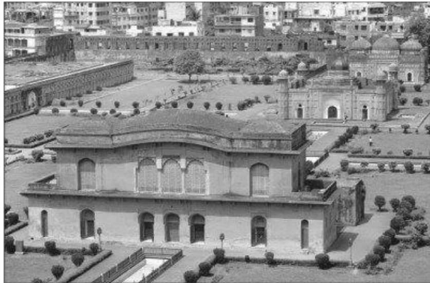
Figure 02: Ground Floor Plan and Aerial View of the Diwan-i-Am of Lalbagh Fort (Source: Unpublished Long Report of the Heritage Studies 2011 , Dhaka Group)
