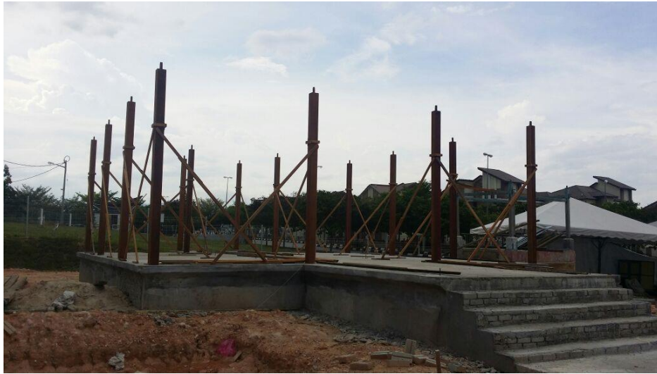
Fig. 3 The reinstalled columns temporarily supported by wooden bracings (Source : ATSA Architects, 2016)
