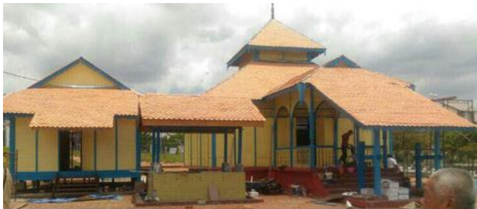
Fig. 6 The nearly completed mosque building and its surrounding (Source : ATSA Architects, 2017)
