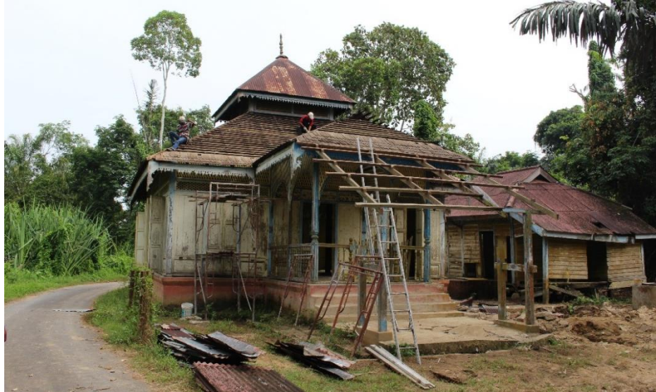
Fig. 2 The dismantling works of the mosque on the old site
