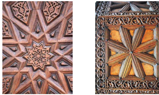
Fig. 9, 10: Window sashes in künde-kârî technique: Before being framed each geometric part is interlocked without nailing, screwing and sticking.
