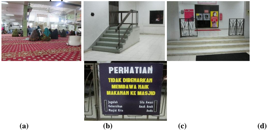
Fig. 3: The safety aspect in MAR: The carpet in the main area inside the masjid (a), the sharp edges on the left wing corridor of the masjid (b), the stairs of the entrance area at MAR (c), and the warning signboard at the masjid (d).
