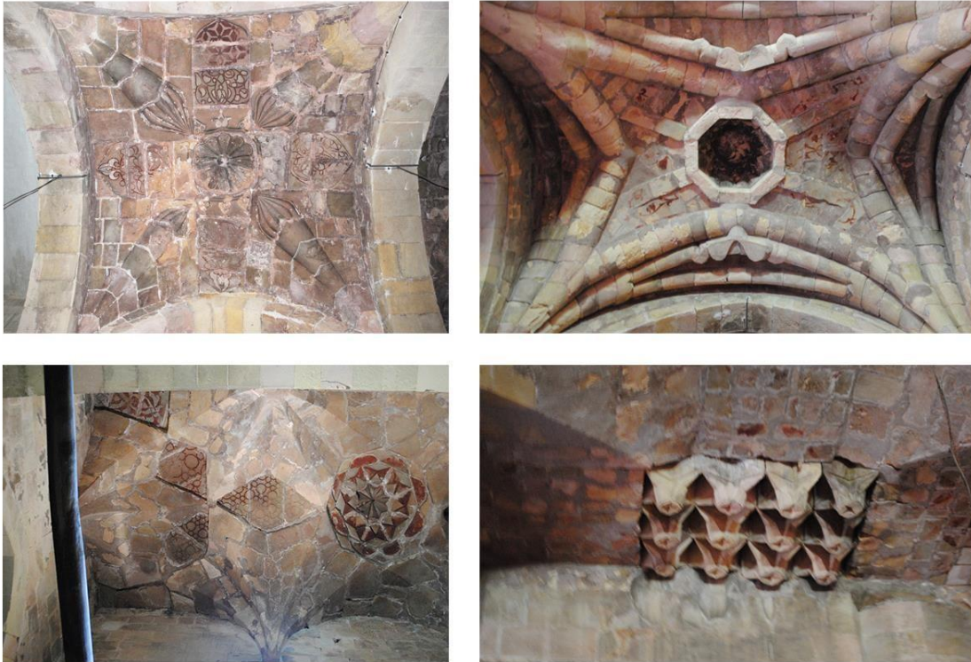
Fig. 3: Cross-vault Stone structures, Great Mosque and Hospital Divriği, Turkey / 2012
