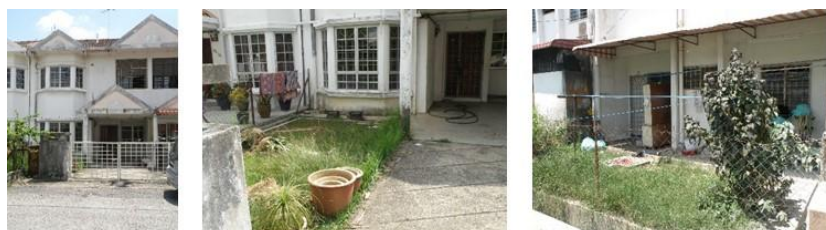
Fig. 4: Typical original front façade of the unit, its front lawn, and backyard
