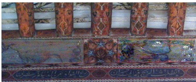
Figure 5: Kube, the ceiling of Iwan, Rami, 2006
