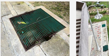
Figure 17: Existing conditions in Courtyard A (Source: Authors, 2025)
