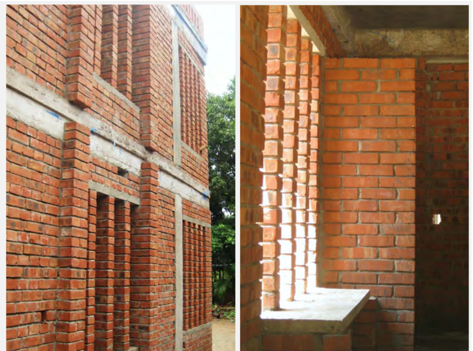
Figure 18: (Left) Slit openings on the west façade from the exterior; (Right) The afternoon sun has been filtered through the slits to protect the bedroom from heat gain.
