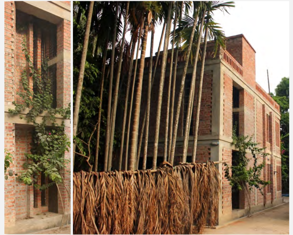
Figure 14: The west façade showing slit openings and vine creeper as a protection from the low altitude afternoon sun.
