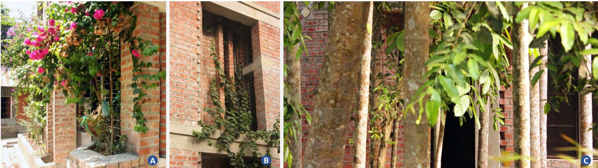
Figure 23: Planting and vegetation (A) at the entrance, (B) on the west façade and (C) north side of the building, enhancing aesthetics and privacy, filtering sun light to reduce thermal gain and blending the house into the context.
