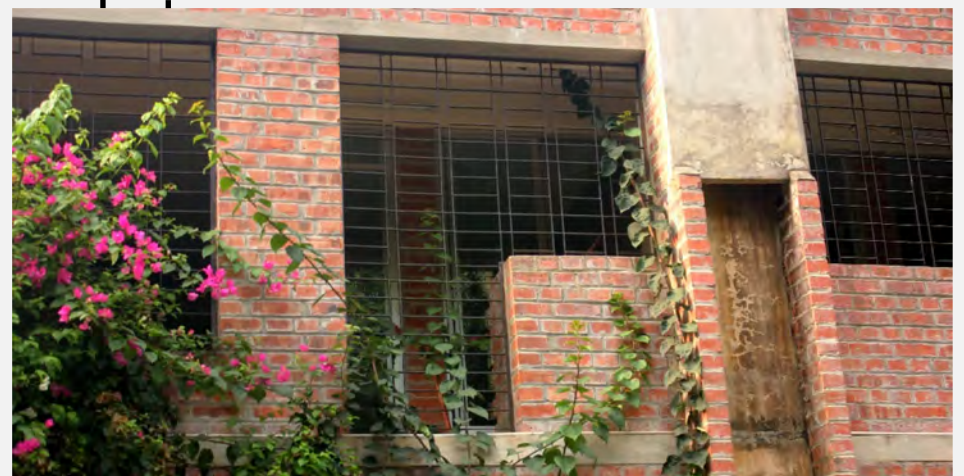
Figure 22: Integrated rainwater spout on the front façade of the building. The water coming down nourishes the bougainvillea plant on the ground floor planter box.
