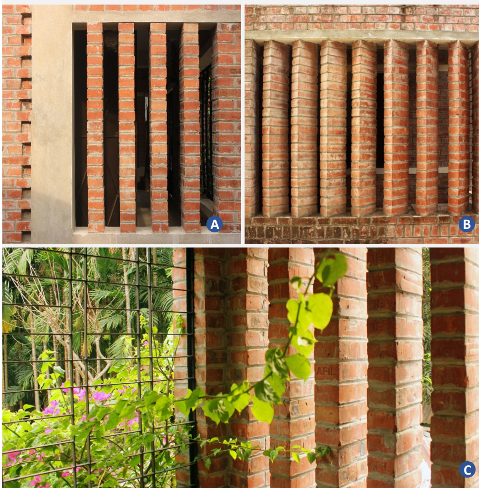
Figure 17: (A) Vertical brick louvre on west façade; (B) Tilted vertical brick louvre on east façade allowing the winter morning sun; (C) Vertical brick louvre on the upper floor veranda providing privacy from the neighbouring houses while allowing ventilation.
