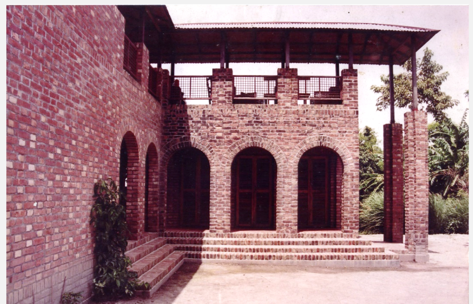
Figure 12: Layered façade to protect the house from heat gain during summer. (Source: Bashirul Haque Architect)
