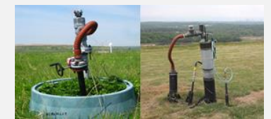
Figure 8: Gas wells on site
