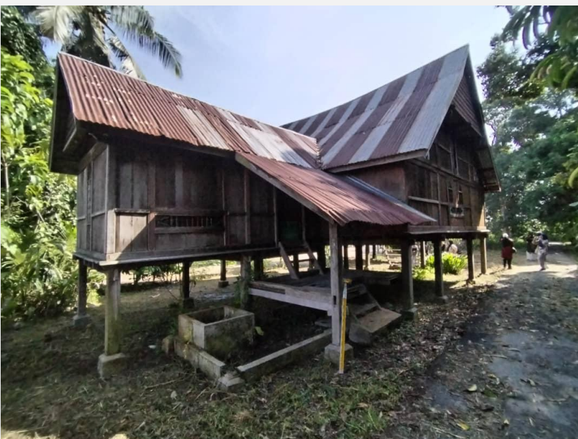
Figure 3: Side view of Rumah Kutai Tok Saudara Bongsu
