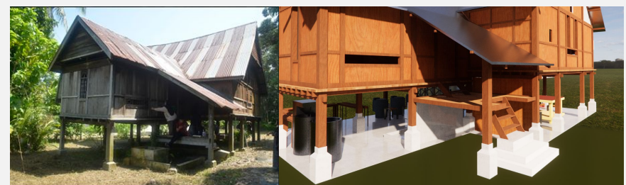
Figure 26: Rumah Toksu's rear facade before rehabilitation (left), after rehabilitation (right)
