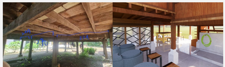
Figure 25: Under house space before rehabilitation (left), after rehabilitation (right)
