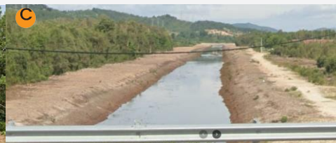
Figure 23: Kijal river near the proposed site. Source: Google Street View
