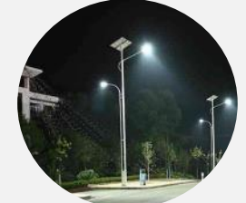
Sensors and Controls
