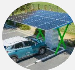
Solar EV Charging
