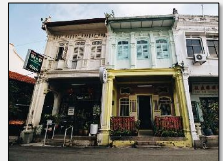
Figure 2: Preserved Commercial Buildings in George Town, Penang (Source: Renée, 2021)
