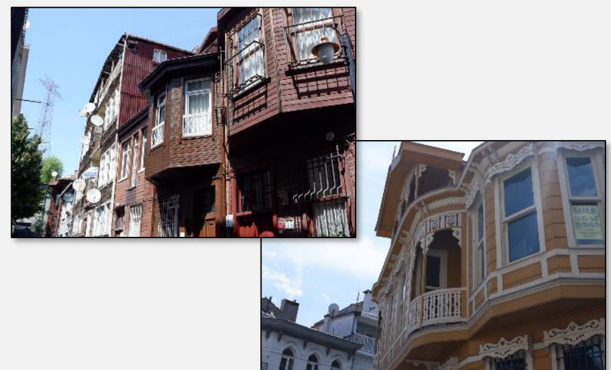
Figure 7: Preserved Residential Buildings in Arnavutköy, Istanbul (Source: Authors, 2023)
