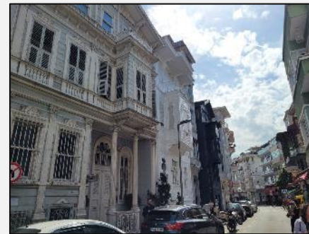
Figure 1: Preserved Residential Buildings in Arnavutköy, Istanbul (Source: Authors, 2023)
