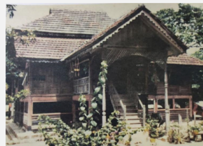
Figure 2: The front view of Rumah Penghulu Haji Abbas before destroyed by a fire in 2003. Source: Warisan Seni Bina Selangor
