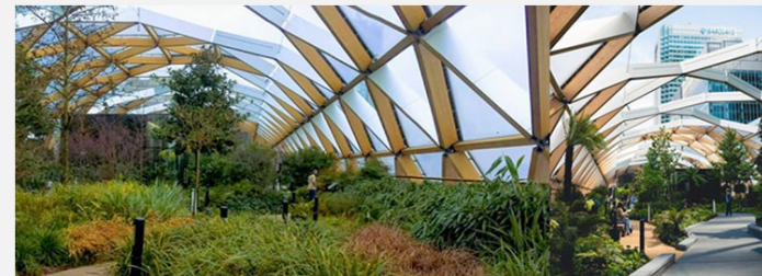
Figure 7 : Cross rail Place Roof Garden
