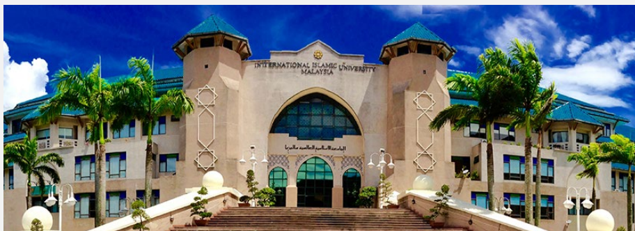
Figure 1: The view of rectory building, IIUM, Gombak (Source: iium.edu.my, 2020)
