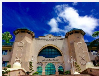
Figure 20: Entrance of rectory building. (Source: GSPBlog, 2016)
