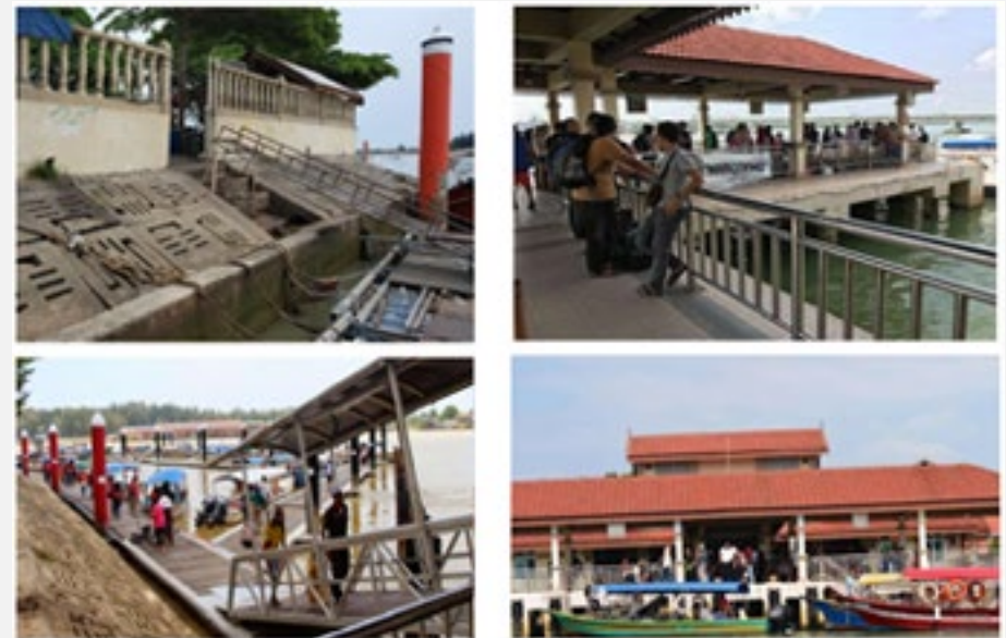
Figure 4: Overcrowding and Safety Concern at the Existing Passenger Terminal and Jetty (Source: Author)
