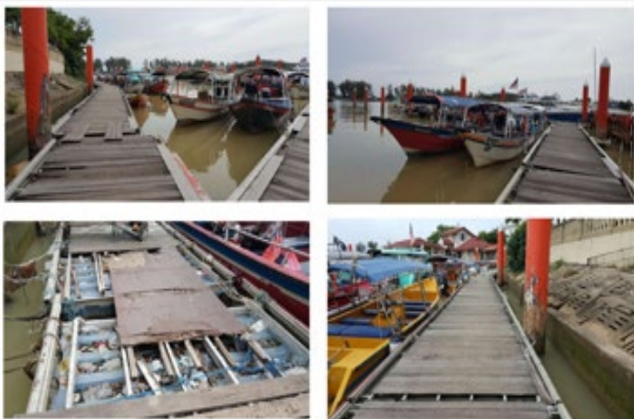
Figure 3: Current Kuala Besut Boat Terminal Jetty Condition (Source: Author)
