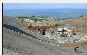
Figure 13.1: Sanitary landfill level 3
