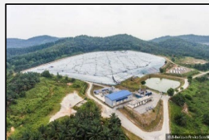
Figure 13: sanitary landfill in Jeram Kuala Selangor
