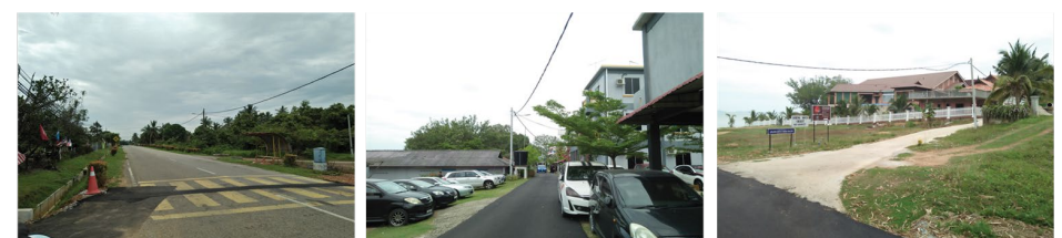
Figure 7: Bad condition of accessibility in Kampung Kuala Linggi
