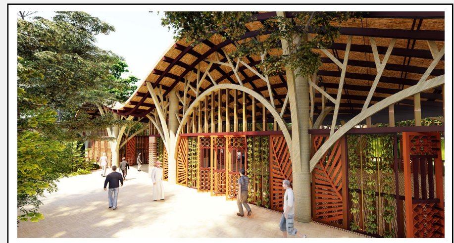
Figure 32: Art & Craft Production building enclosed with decorative wall panels made from plastic waste
