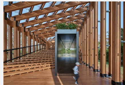
Figure 5: Growing Up public pavilion in Hong Kong (Source: freight.cargo.site)
