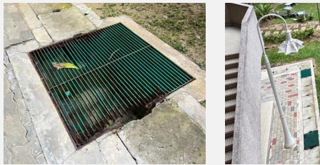
Figure 17: Existing conditions in Courtyard A (Source: Authors, 2025)
