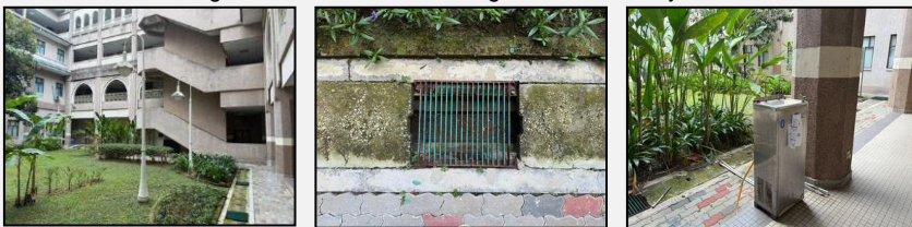
Figure 14. Figure 15. Figure 16. Figure 14,15, and 16 Existing utilities at Courtyard B
