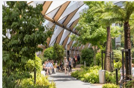
Figure 8: Crossrail Place Roof Garden's Multifunctional Green Roof Strategy (Source: Google)
