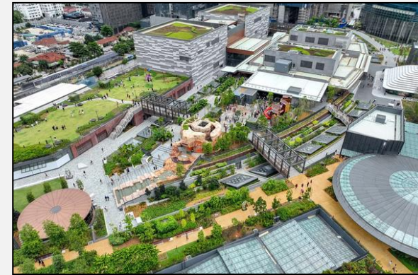
Figure 5. Aerial view of TRX City Park.
