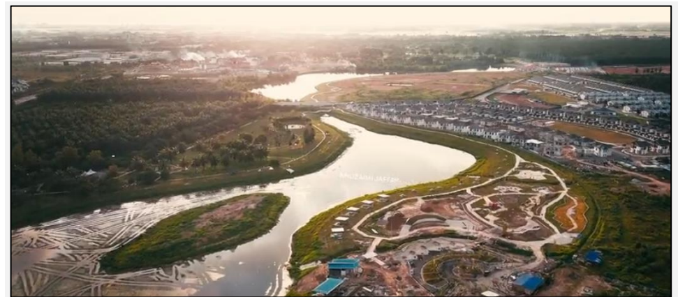
Figure 34: Aerial View of Current Bertam Lake park
