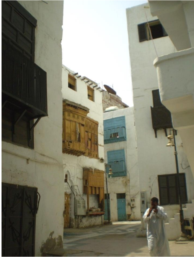
(A residential area in the old city of Jeddah, Saudi Arabia)
