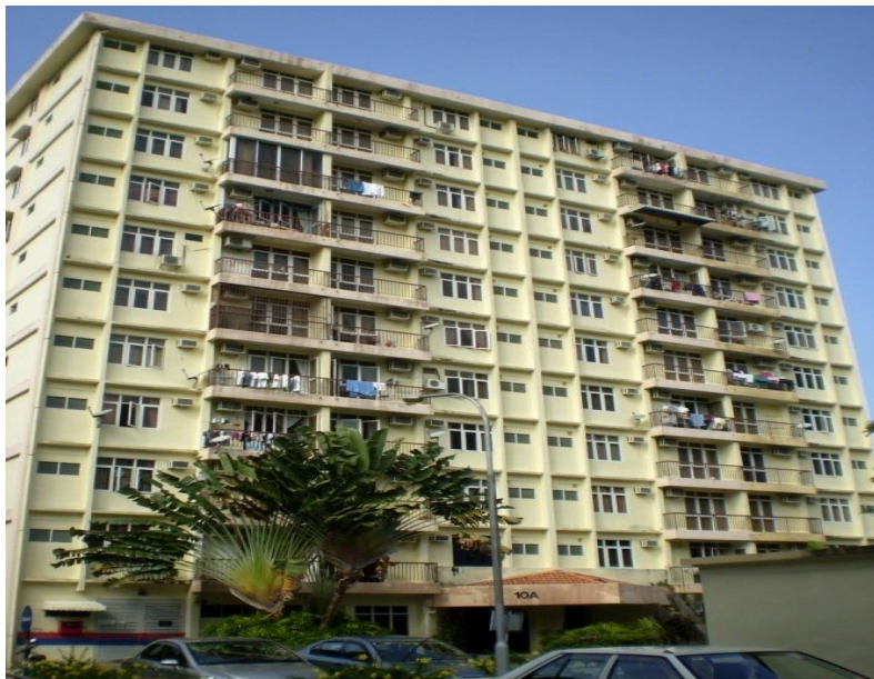
An apartment building in Penang, Malaysia.
