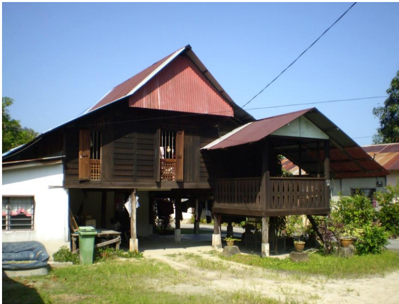
A village house in Penang, Malaysia.
