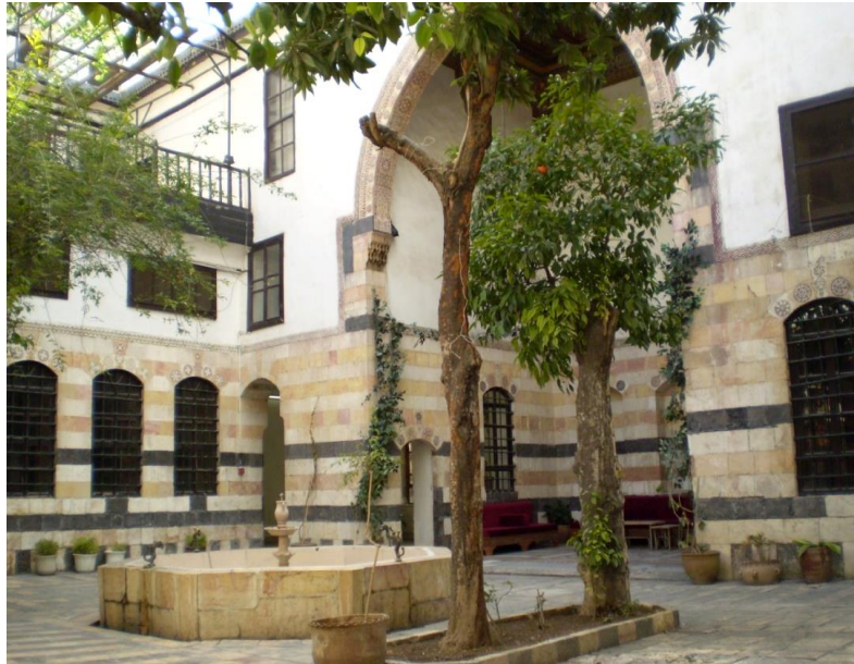
A courtyard house in Damascus, Syria.
