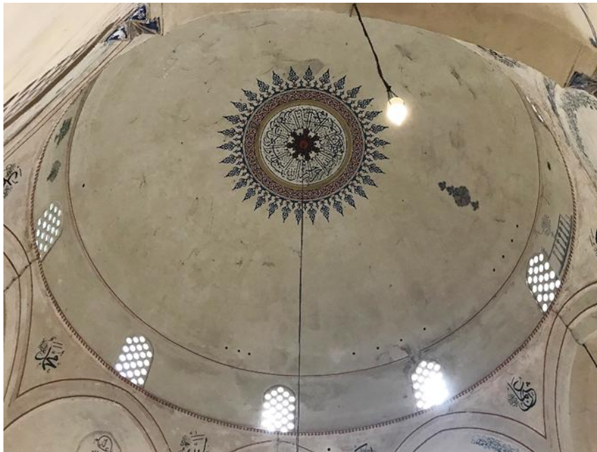
Figure 3. An abundance of natural light permeates the mosque's interior through 25 sizable windows. Eight of them pierce the drum of the dome.
