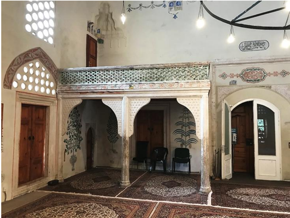
Figure 5. The mahfil and the entrance at the rear side of the mosque.
