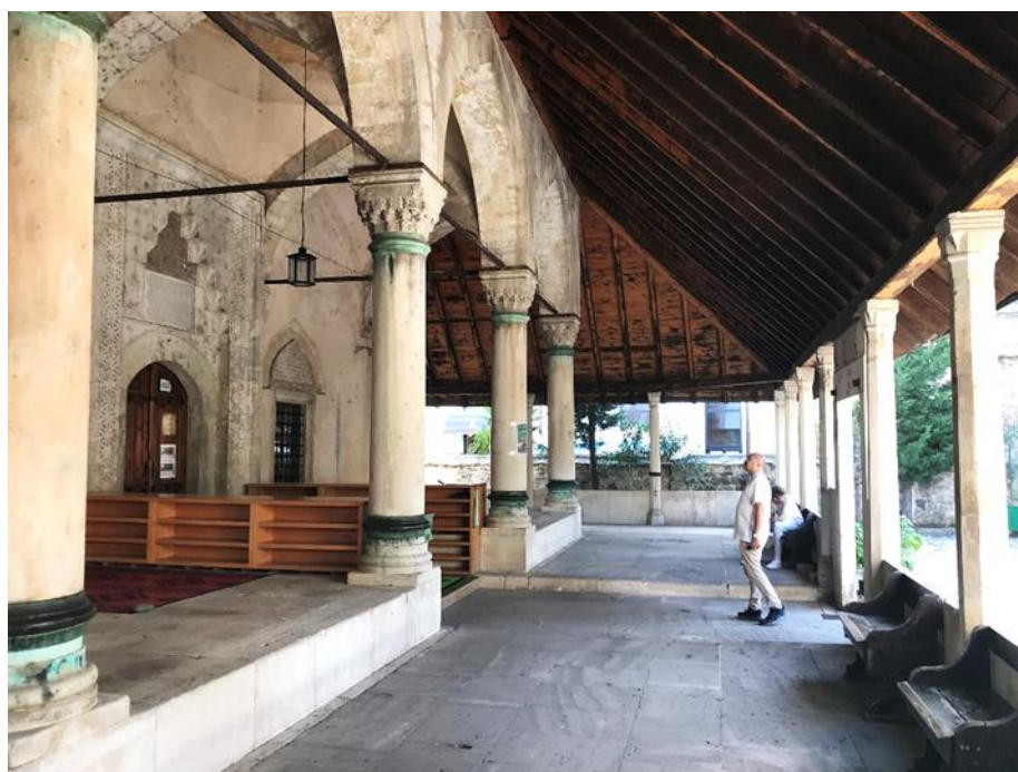
Figure 6. The mosque comprises a two-part frontal portico: an inner domed section adjoining the prayer hall and an outer section sheltered by a steeply pitched wooden roof.
