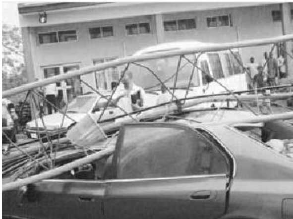
Figure 4: A mast fell on a car, destroying the car and probably killing the occupants 51
