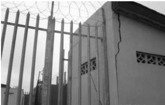
Figure 2: A mast site at Idofian, Ifelodun LGA, Kwara State showing the cracked wall of the Plant Room of the Base Station as a result of vibration from its generators. 35
