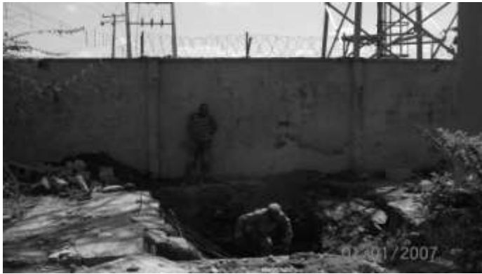
Figure 3: A collapsed septic tank at No 13 Sadiq Sulyman Street, Fate, Ilorin, Kwara State, Nigeria due to vibration of power generator in a close by telecom Mast site. 36
