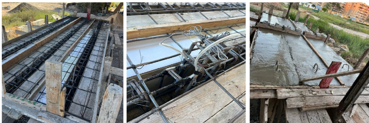
Figure 2. Fabrication stages of the tested continuous RC beam specimens.
