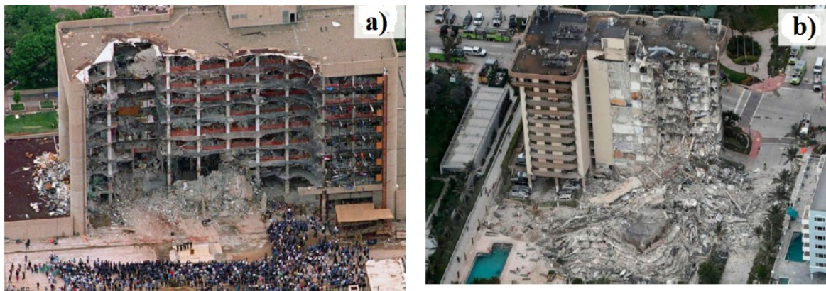
a) Collapse of the A. P. Murrah Building [24]
