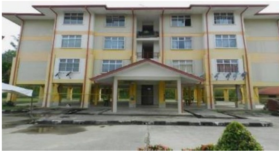
Figure 3. Front view of staff quarters of SMK Ranau.
