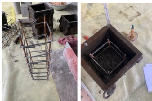
Fig. 3: Steel reinforcement of RC columns.
