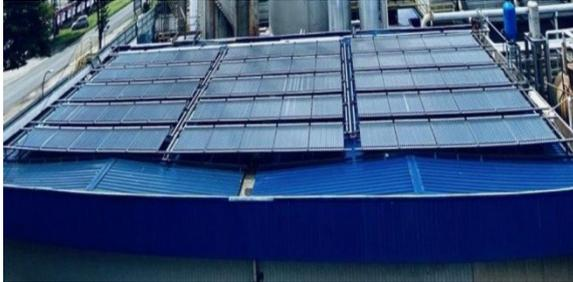
Fig. 1: Array of Evacuated Tube Collectors (front view).
