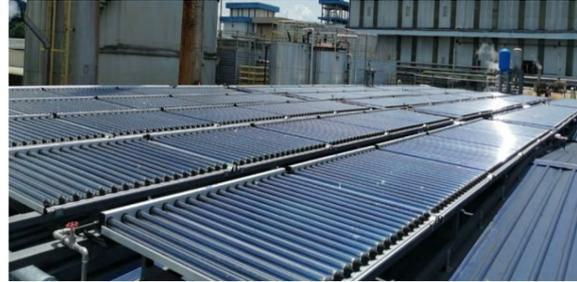
Fig. 2: Array of Evacuated Tube Collectors (side view with 10 degree inclination).
