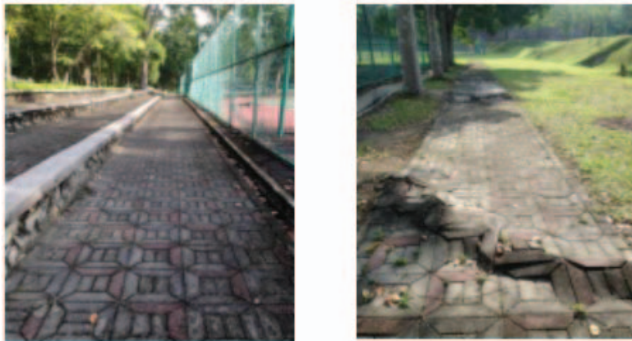
Fig. 4: Smooth pavement (left) and uneven pavement with irregularities (right).
